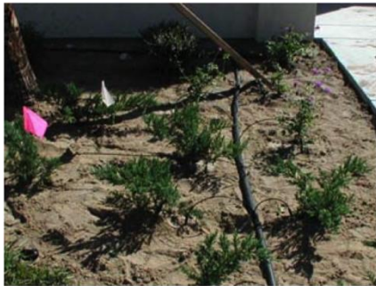
Figure 4. Individual drip emitters.
