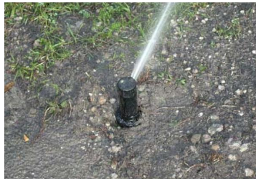
Figure 2. Gear-driven rotor irrigation head.
